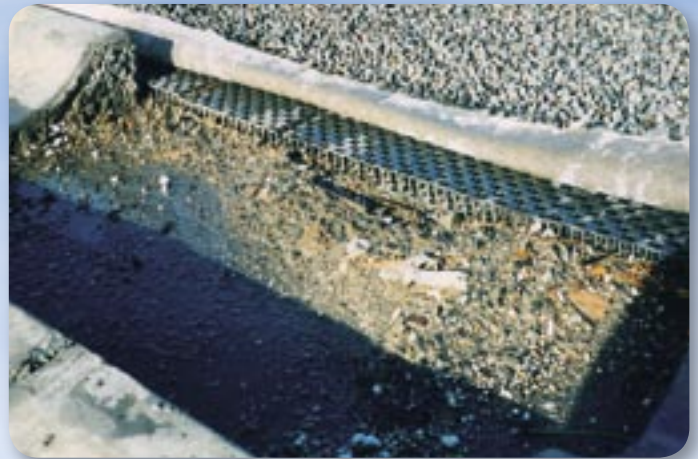
View of Atlantis® Drainage Cell beneath road base.
