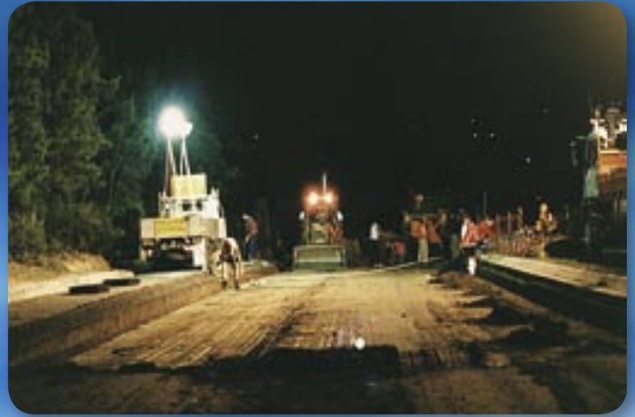
Excavation of road and removal of previous drainage system.
