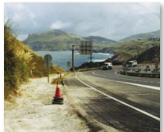
Completed installation, Valencia Spain.
