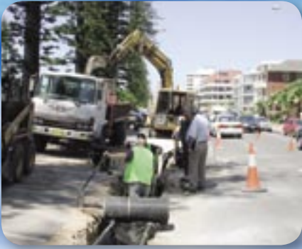
Installation of Atlantis road system at Manly Beach, Sydney, NSW.
