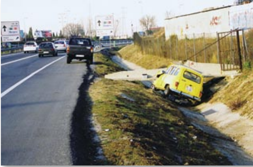
Over a thousand people die on Spanish roads every year due to road drainage design.
