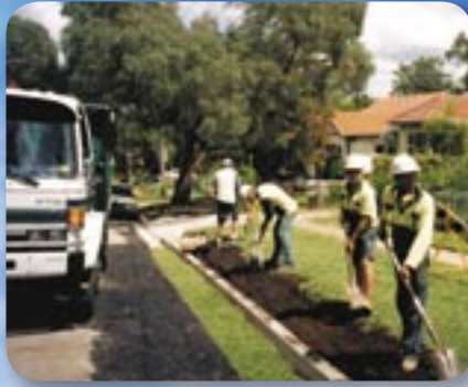
Installation of Atlantis road system at Concord, Sydney, NSW
