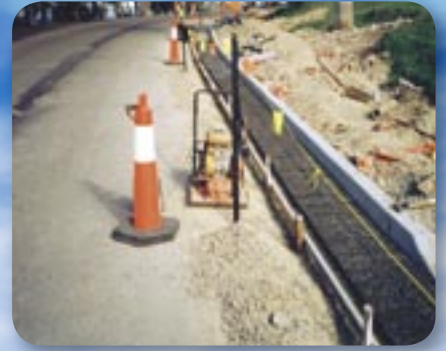
Installation of Atlantis road system at Lake Macquarie, NSW
