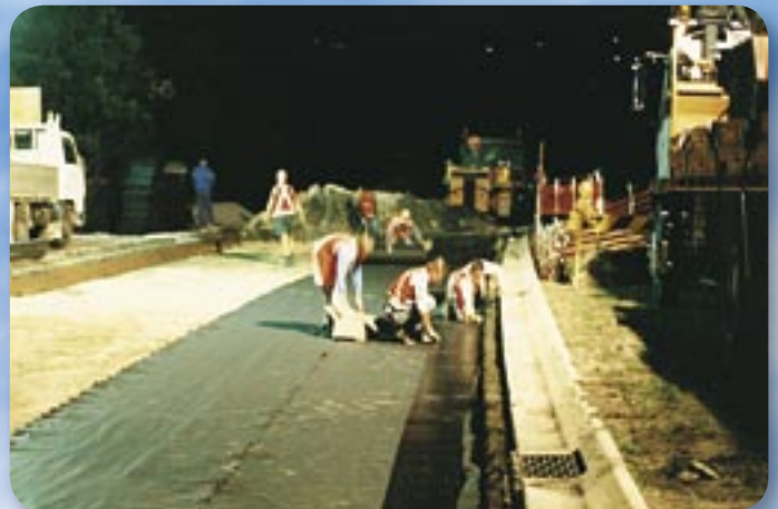
Installation of geotextile being laid over Atlantis® Drainage Cell.
