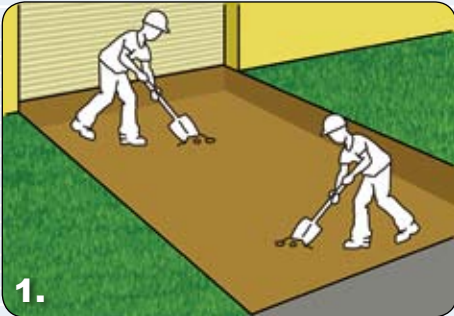
1. Excavate the area out at approx. 250mm of depth. Base of excavation should be flat and relatively level.
