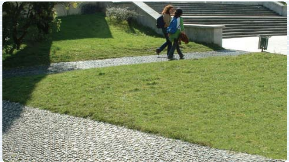
Gravel Cell® reinforcement structure installed for pathways on a university campus.
