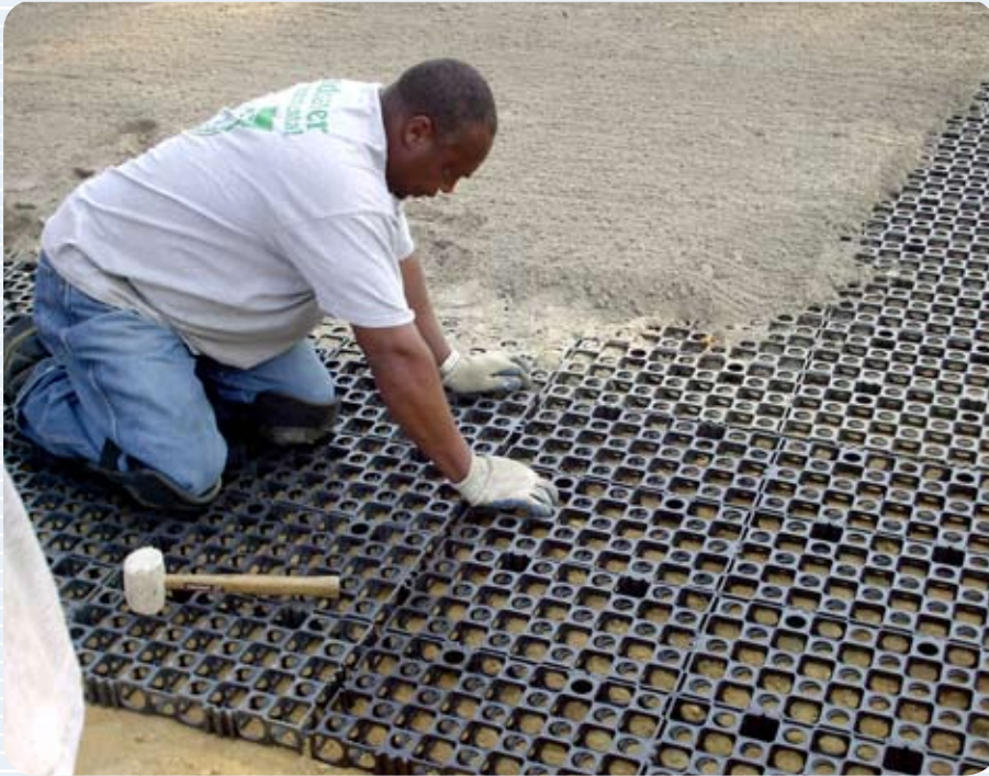
Gravel Cell® reinforcement structure installed for pathways on a university campus.
