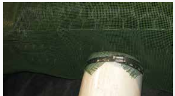
Figure 18: Cut "X" in Biaxial Mesh and Geotextile to accommodate outlet pipes and seal with stainless steel band clamps
