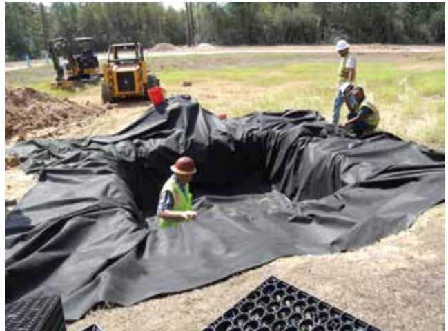
Figure 6: Roll out geotextile cut to fit the excavation in order to keep in-situ soils from migrating into the FocalPoint System. Geotextile strips must be cut generously in order to cover entire excavation on completion of the installation.
