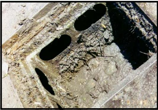
The picture to the left shows the **Grate Inlet Skimmer Box** immediately after the removal of booms and skimmer tray. Notice the bypass openings around the top are completely unobstructed. The filter is full to capacity and is operating in bypass mode. Because this inlet experiences an extra heavy hydrocarbon pollutant load it is fitted with extra **Storm Booms**.
