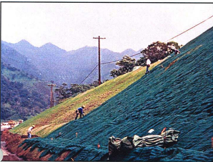
This site presented major aesthetic challenges in preserving this breathtaking Oahu Landscape (right). Landlok® TRM 435 is installed on a moderate slope (above).
