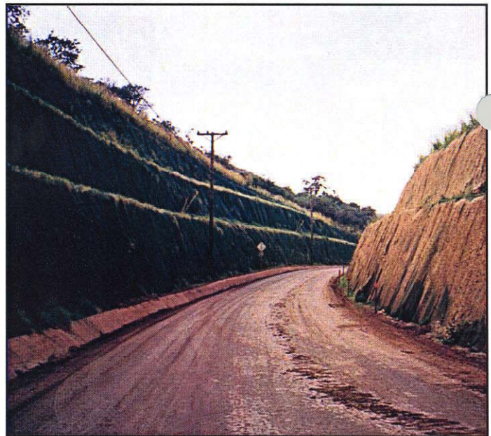
Landlok® TRM 435 used to limit weathering and raveling of rock cuts
